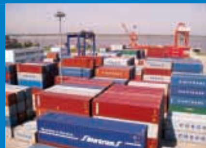
WIT Port in operation
