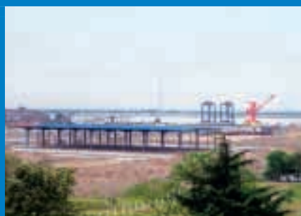
Construction of the WIT Port in progress
